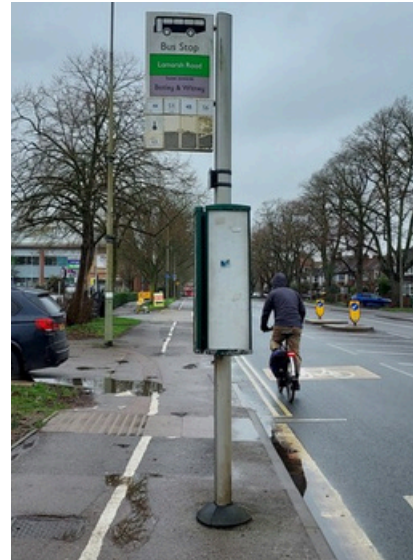
This is substandard provision. Note the bus stop in the bike path
